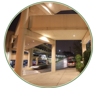
After energy-efficient retrofit
