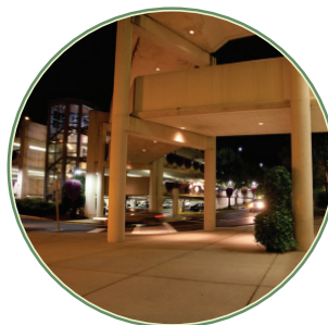
Before energy-efficient retrofit
